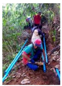
constructed, before 3.5km of pipes were laid from the water source to the site of the storage tanks. The two 10,000 litre tanks were then constructed above the village allowing a combination of gravity and water pressure to deliver water around the village. After completion, a network of pipes were laid and 12 standpipes with taps were installed.
